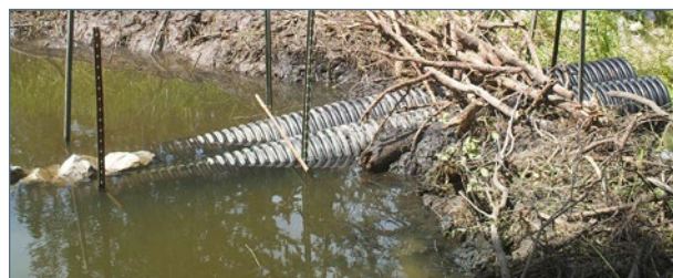
Pond leveller installed at Piper Creek (BELOW)
